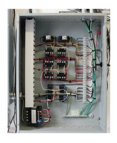
enclosures because of the greenhouse environment. CropKing uses only UL listed components, however some codes require that the constructed panel be UL listed. In some areas, agricultural buildings are exempt from electrical zoning. Please check with your local electric codes.
