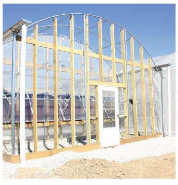
**THE SOUTH END WALL** is framed using locally purchased heat-treated 2"x4" or 2" x 6" lumber and covered in twin-wall polycarbonate that is part of the greenhouse covering package. Alternatively, the south endwall can be framed with steel purchased from CropKing, but we often find it is more economical for the grower to frame the endwalls in locally purchased, heat-treated lumber.
