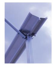
during polycover installation. The extrusion contains a quicklock base so the quicklock cap can be locked in place to secure the polycover. This polylock package makes the installation and replacement of the polycovers simple.
