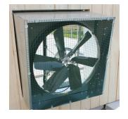
**THE EXHAUST FANS** are manufactured by American CoolAir, a renowned manufacturer of agricultural fans. 2 exhaust fans with slope wall housing are located on the north endwall of each bay. Air is pulled from the south end of the greenhouse through American CoolAir's evaporative cooling system and pushed out through these fans.
